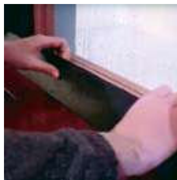
The cover profile is easily clicked open.
