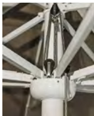
TIG-welded aluminum rib port collars
